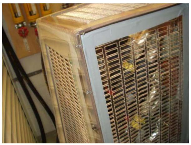
Figure 7-2 Example of a protective cover for the motor connection
